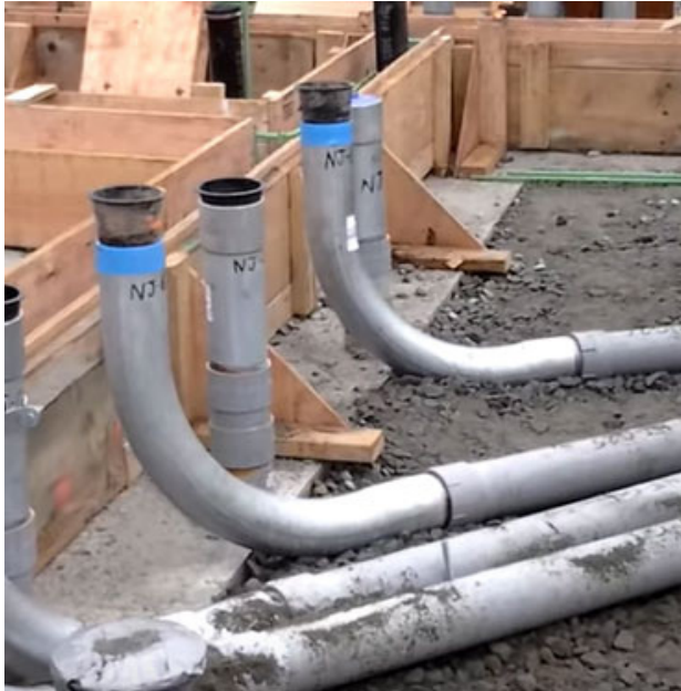
PVC Conduit Stubbed-Up with GRS Elbows
